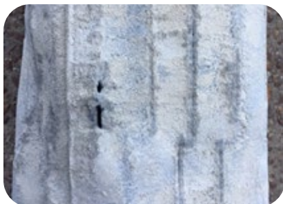
BEFORE – Frequent Failed Filter Bags
