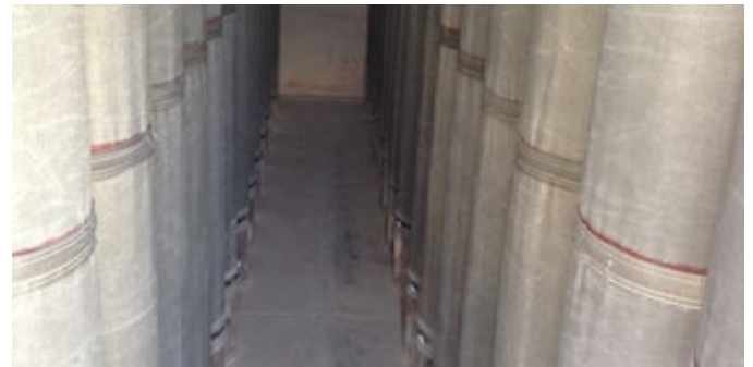
Finished Installation. Filter Bags at Tension
