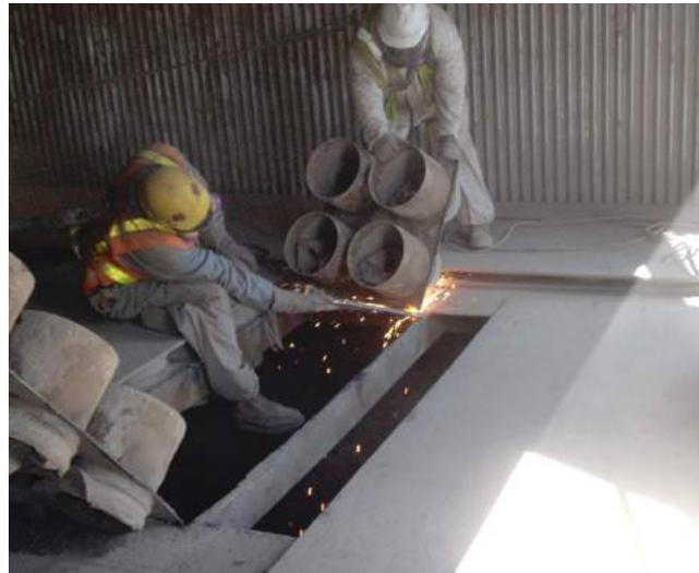
Eliminating thimbles from the tube sheet
