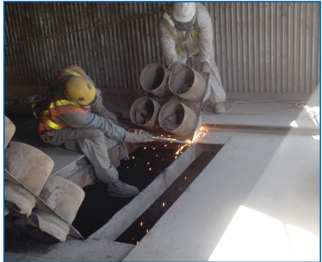
Eliminating thimbles from the tube sheet
