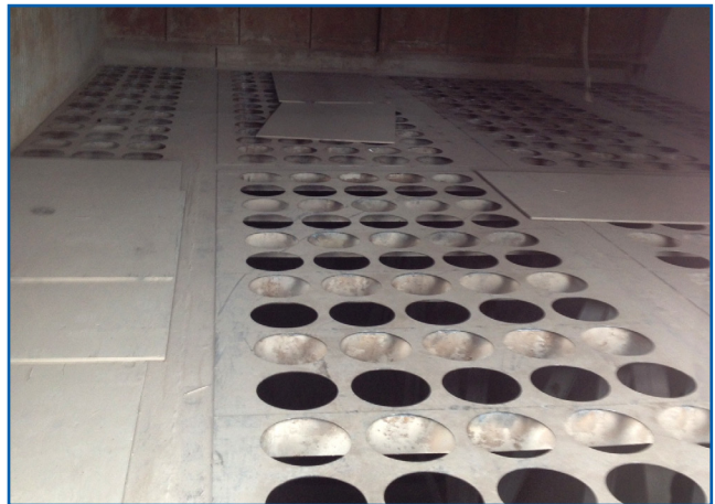
Converting to new, snapband style floor
